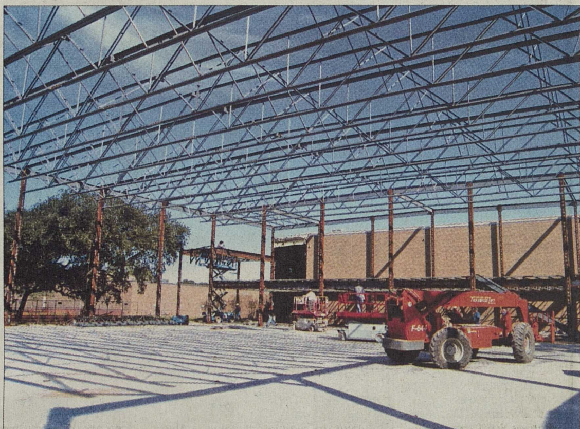
The frame of the new gym for the Rice Junior High is on its way up in Altair.
